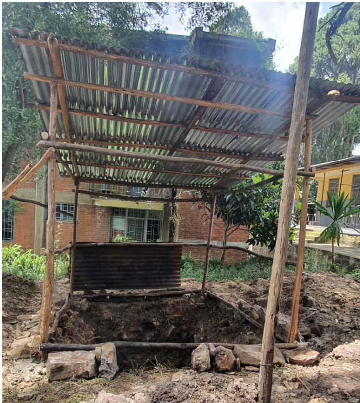
Newly built solid waste disposal site at quarantine facility.
